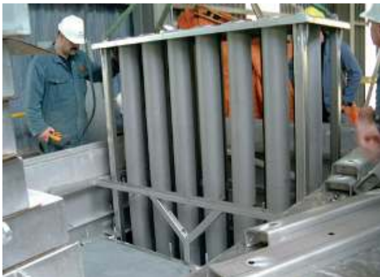
Installation of filter elements.
