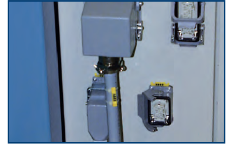
Plug connector for connection to a process data system
