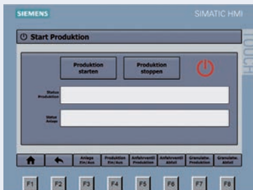
Start of the pelletizing process at the push of a button
